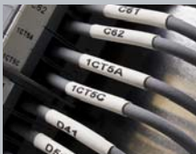
Wire & Cable Labeling
