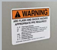
Arc Flash Labeling
