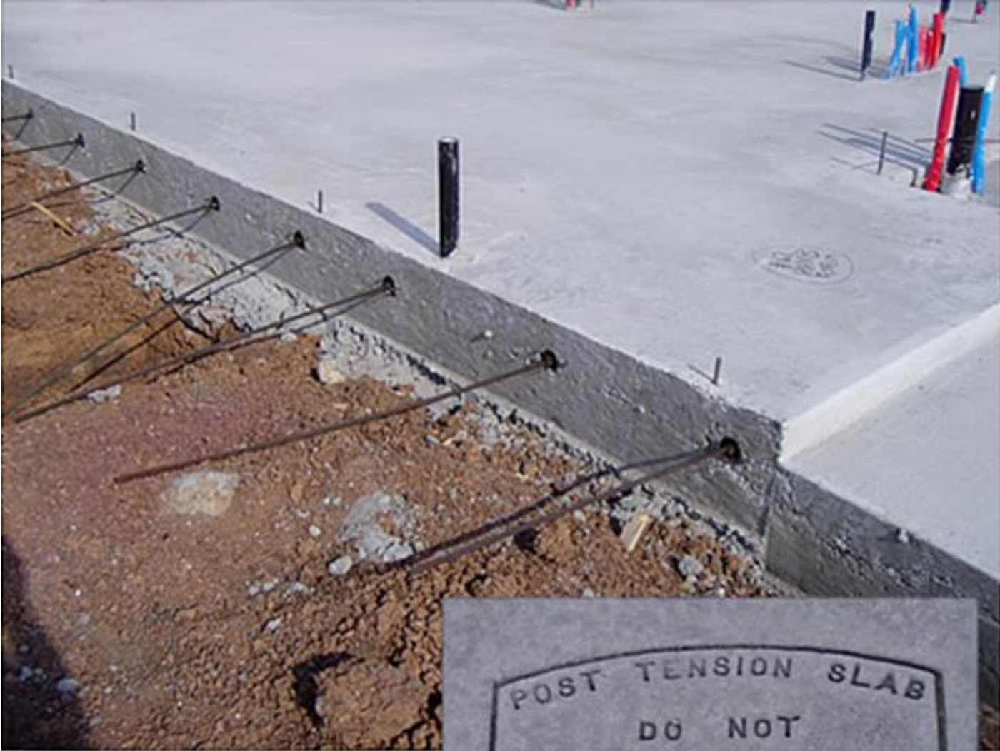
Post Tensioned Slab
