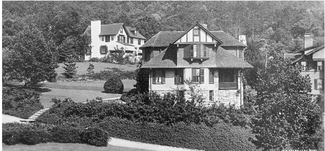
Very little grading was done to accommodate the cottages in the landscape of Albemarle Park.
