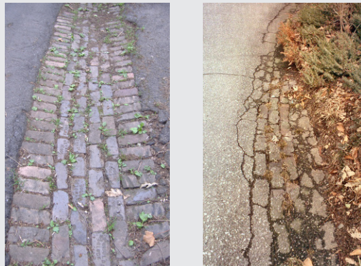
(Below) The brick drainage swales throughout Albemarle Park were covered over with asphalt.
