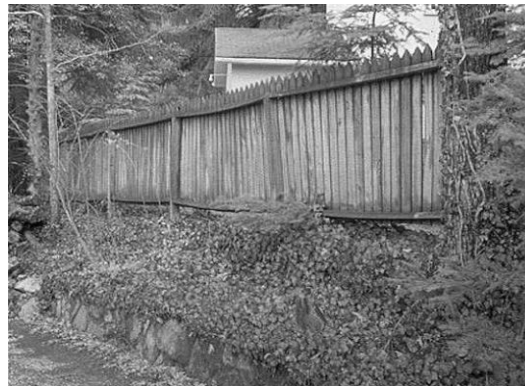
Fences that create a complete visual barrier are discouraged, except in certain areas along the perimeter of Albemarle Park, where such fencing was once used. A mixed arrangement of plantings can achieve the same goal of visual privacy.
