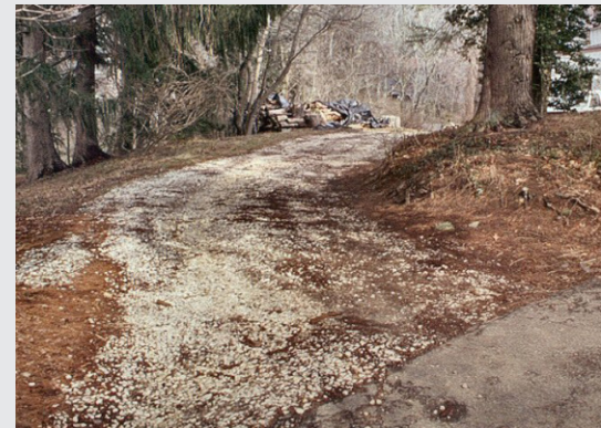
(Below) Loose white gravel was used as driveway paving material in several areas.
