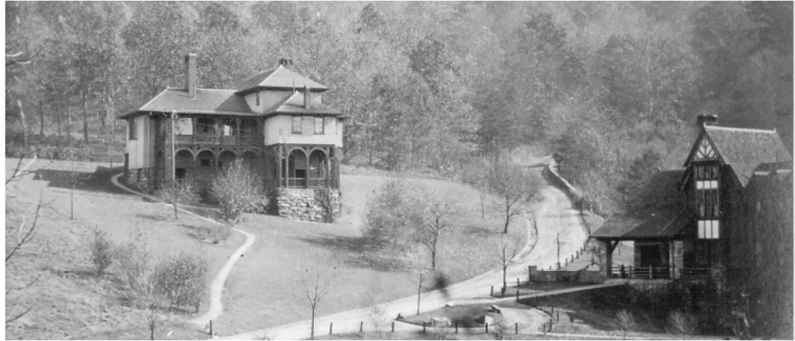
A fundamental element of Samuel Parsons' design is its open, shared landscape. Cottages are situated on the land, not to be solitary dwellings in their own private enclaves with front yards and back yards, but, rather, parts of a resort park campus, a 35-acre planned community in which the buildings and the landscape complement one another.
