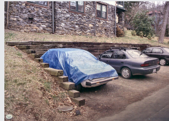
(Above) Bank along Cherokee Road was excavated and buttressed with railroad ties to provide parking.
