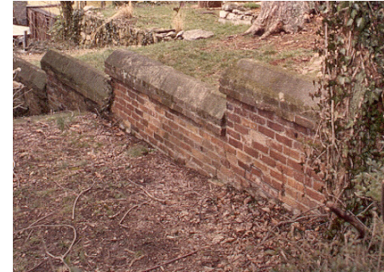
Brick was used for low retaining walls in several places.
