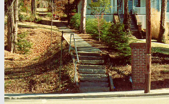
(Above) The steps at the foot of Hillside Walk in 1989.
