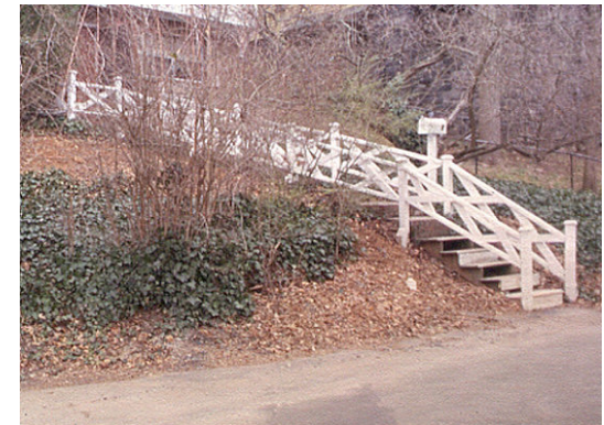
Fences and railings should blend into the overall landscape. In this case, a more appropriate design would utilize a simple iron pipe rail.
