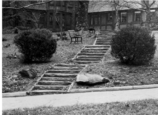
After the original wooden steps used in Albemarle Park likely rotted away, more durable steps were created using large granite blocks, as in this area of the front lawn of The Manor Inn.
