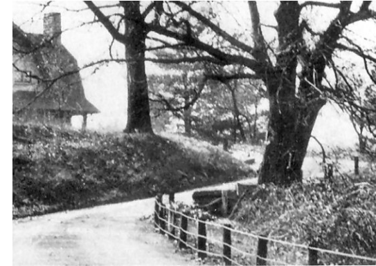
In some instances, one to three cables were strung between the log bollards to create a fence. This view shows the fence in the bend of Orchard Road just above the turret at the southeast corner of the Clubhouse.
