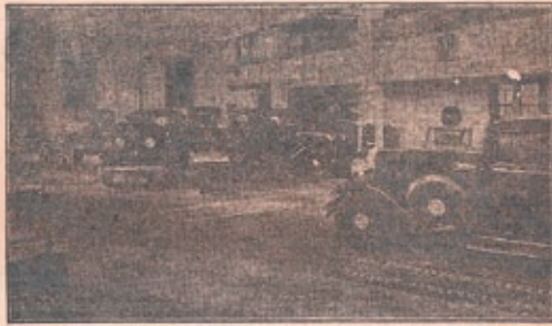
Attractive showrooms of Pike Motor Corporation, 612 Culver Road
