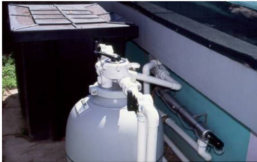
Three types of filtration- Mechanical (Grey pond filter), Biological (black tub with dense matting) and UV Clarification/Sterilisation (Stainless steel tube)
