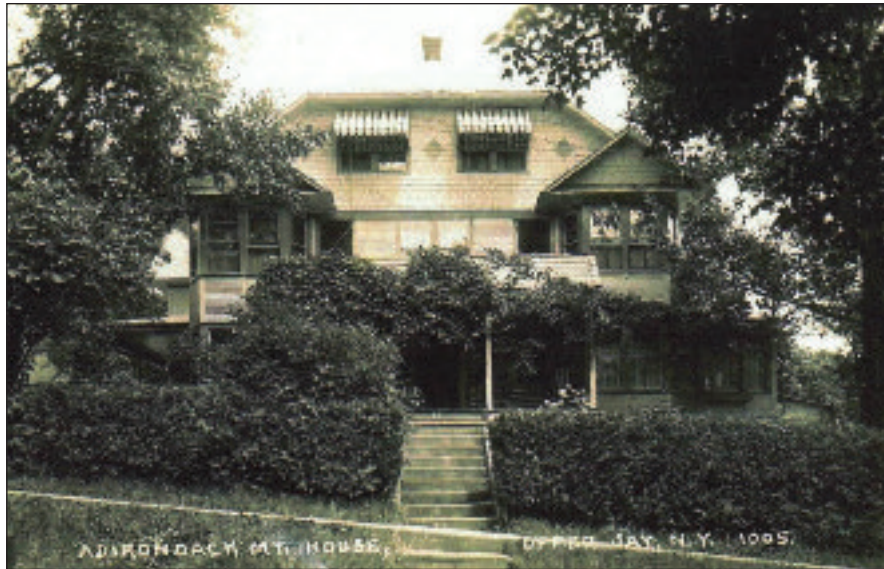
The Adirondack Mountain House overlooked the East Branch of the Ausable and catered to anglers from the 1920s into the 1940s. Photo used with permission of Wells Memorial Library, Upper Jay, N.Y.
