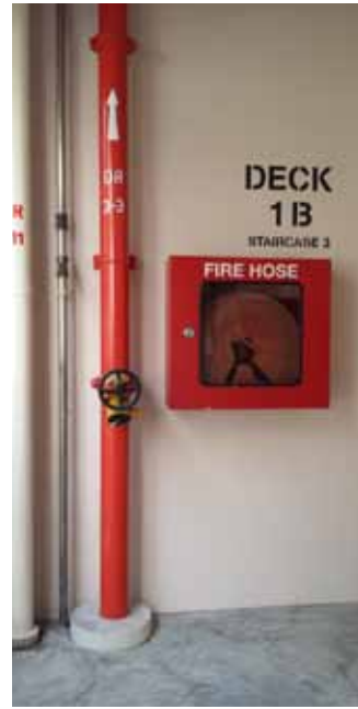
Unobstructed dry risers.
