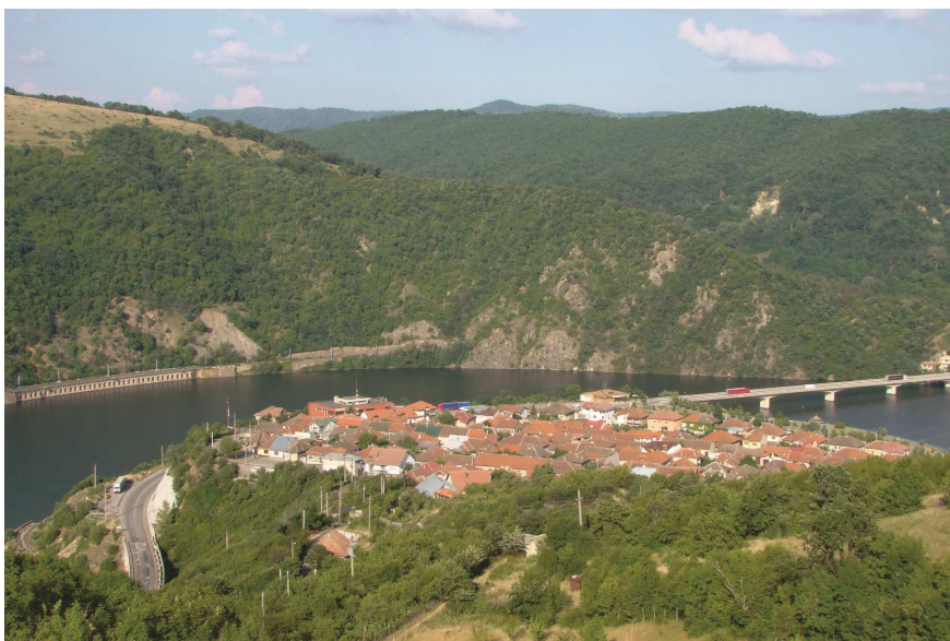
Fig. 14. 140-160 m terrace in the area of the viaduct over Cerna Gulf
