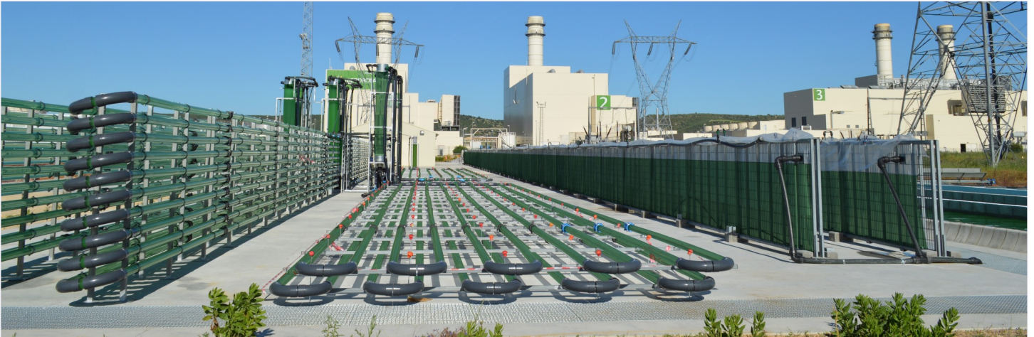
Figure 6: General view of the production plant in Arcos de la Frontera. Vertical Tubular PBRs are shown on the left, Horizontal Tubular PBRs are placed in the middle and Vertical Flat Panels are shown on the right of the photograph. At the back, the Combined Cycle Power Plant belonging to Iberdrola (1.6 GW of installed capacity) is shown.
