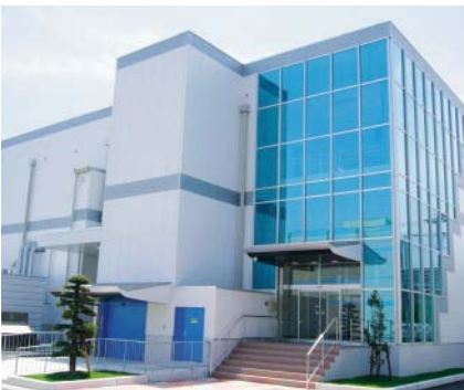
Large-pellicle plant, in Nobeoka.
