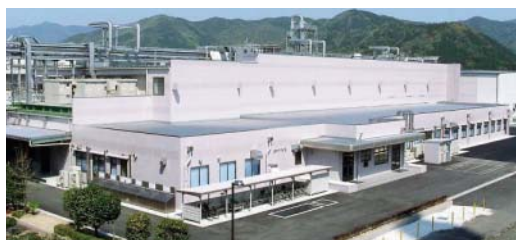
Polysulfone hollow-fiber membrane spinning plant, in Nobeoka.
