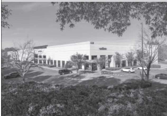
Still in full swing: the relocation of the commercial departments of Oerlikon Textile Inc has already been completed, so that the customer support can already be provided at the new location in Charlotte, North Carolina. The mechanical repair workshop and the electronic repair workshop will follow in the coming months.
