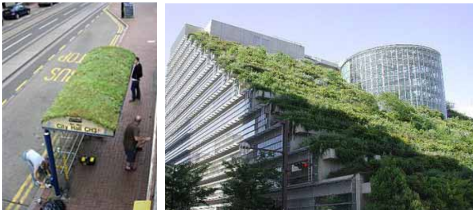
Figure 17: Structures responding to stormwater management . Images left source www.greenroofs.com
