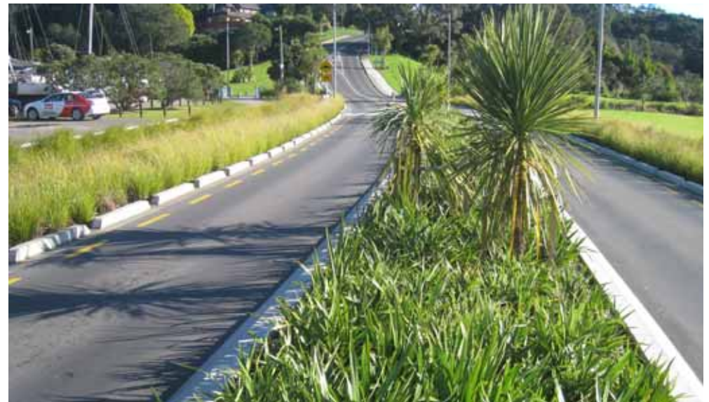
Figure 29: Raingardens enhance the street amenity while also giving cues for slower vehicle travel
