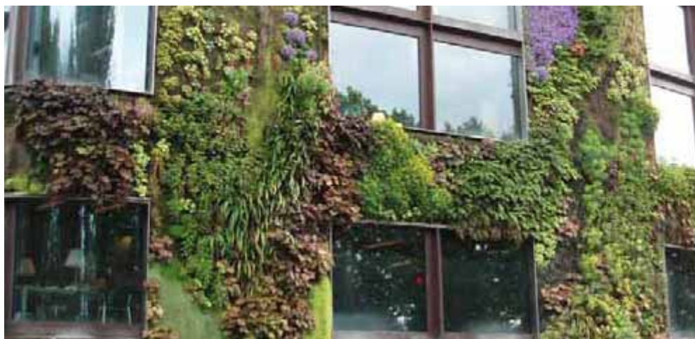
Figure 27: Green walls provide further visual and ecological diversity to city environments and opportunities to capture and treat stormwater
