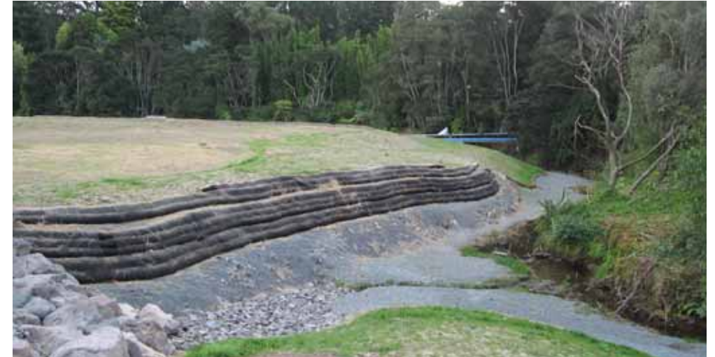
Figure 19: Biotechnical approaches to channel and bank stabilisation, provide the means to support plants based systems
