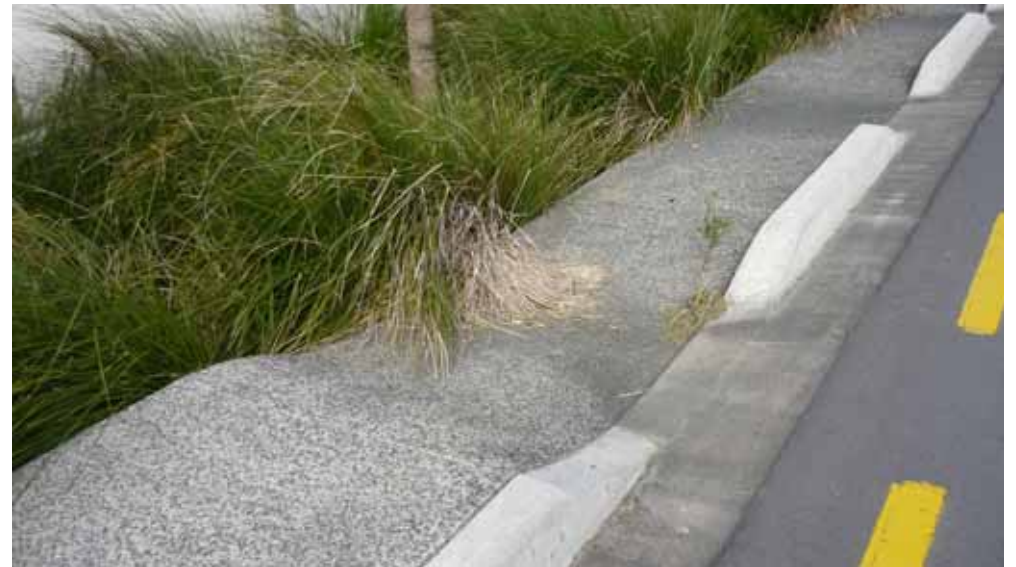
Figure 37:As part of a maintenance programme, make sure planting is not forming an obstruction to stormwater inputs
