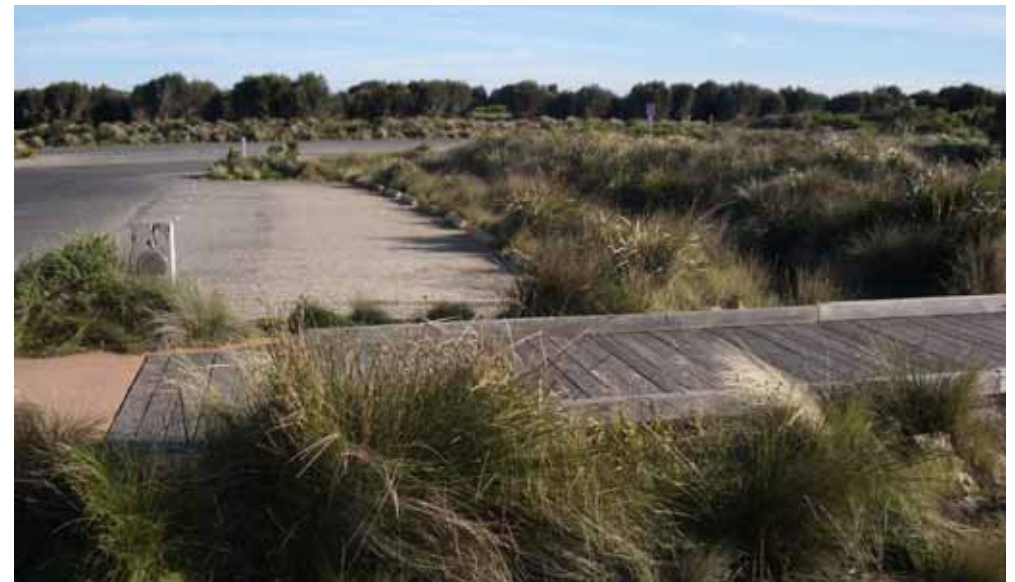
Figure 35: Pedestrian structures provide access over raingardens and an opportunity to view planting
