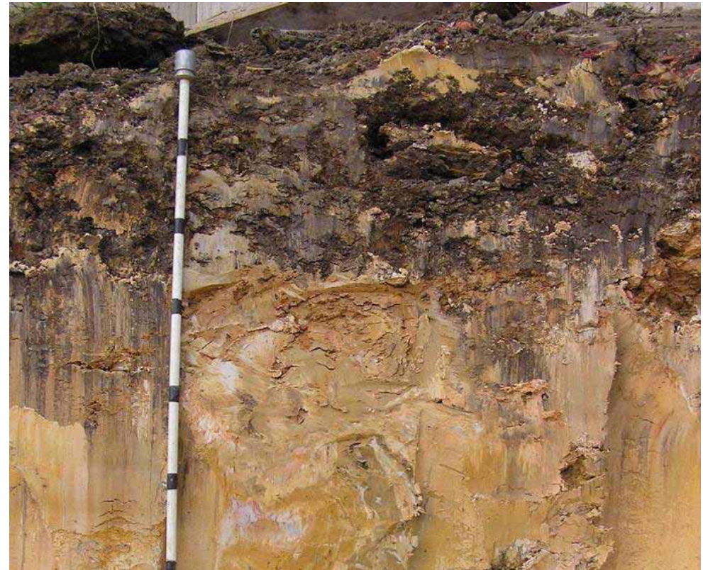
Figure 22: Ultic soils following compaction
