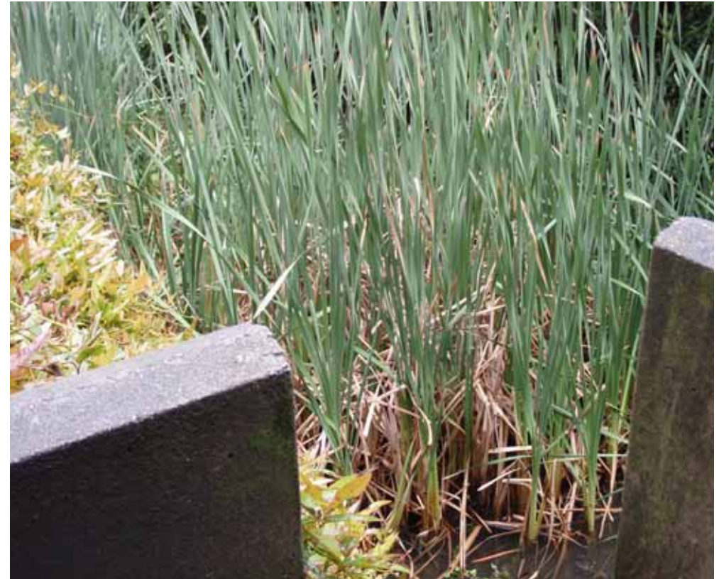
Figure 8: Concrete gaskets contain stands of raupo, which are a highly effective plant for the removal of sediment from stormwater, but are often likely to spread and dominate wetland areas
