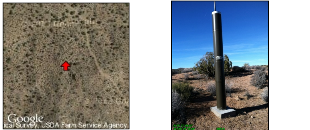
Photopoint 015. This element of the Mohave County Alert Weather System was recently constructed about 100 feet west of BLM Route 7849.
