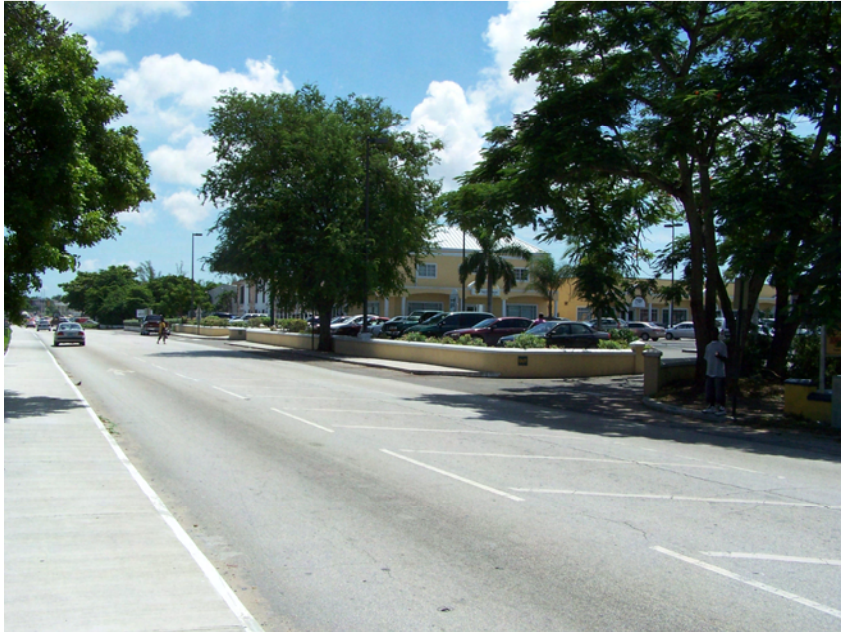
Figure 4.9 Developed Eastern end of project looking south east
