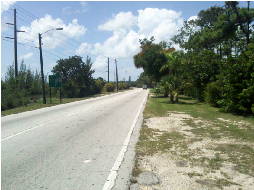
Figure 4.8 JFK Drive east of Blake road looking west
