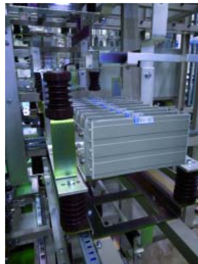
Figure 4: Semiconductor fuses rated at 10kV - 1000 A with low inductance
