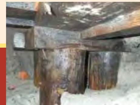
Excavated foundation piles in Amsterdam.
