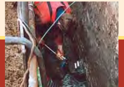
Foundation inspection pit in Haarlem (the Netherlands), piles are measured and sampled.
