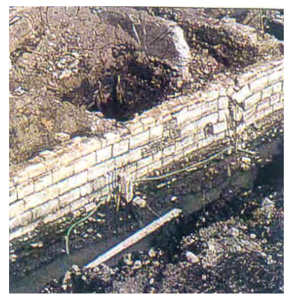
Figure 56c: The long wall of Istria stones, with its foundation piles beneath, dating 16 th century, found on the island of Giudecca .
