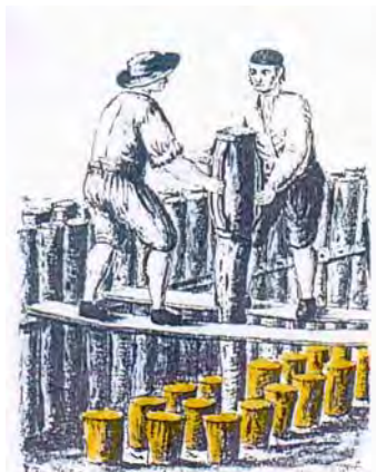
Figure 58a. A system for driving wooden poles by hands.
