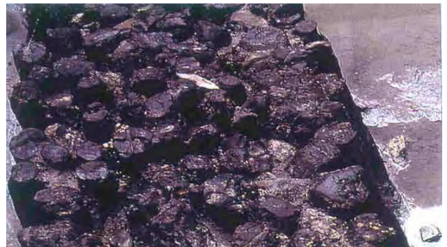
Figure 53b: The row of piles is made of small logs 8 to 16 cm width.
