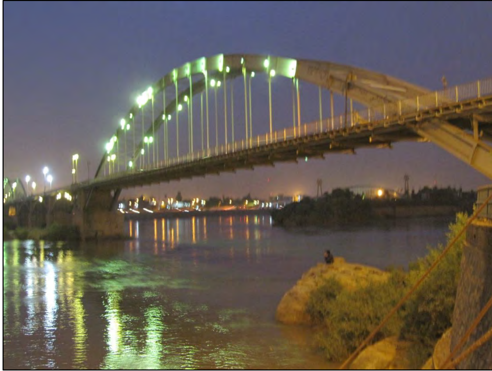
Khuzestan, Karun River at Ahvaz White Bridge (Iran – Ahvaz White bridge^ Karoon, CC BY 3.0, Alireza Javaheri).
