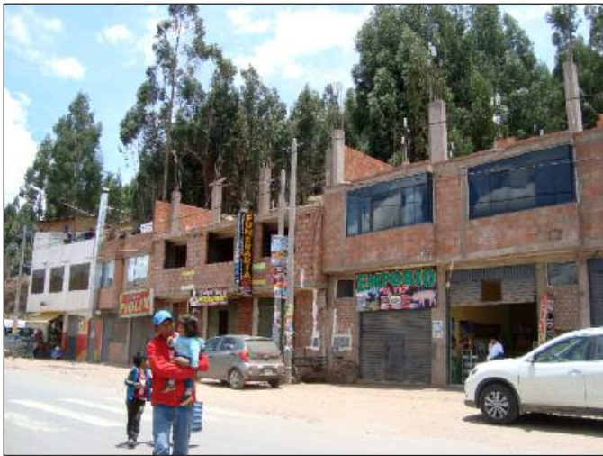
Figure 17. Inhabited buildings still waiting for another storey.
