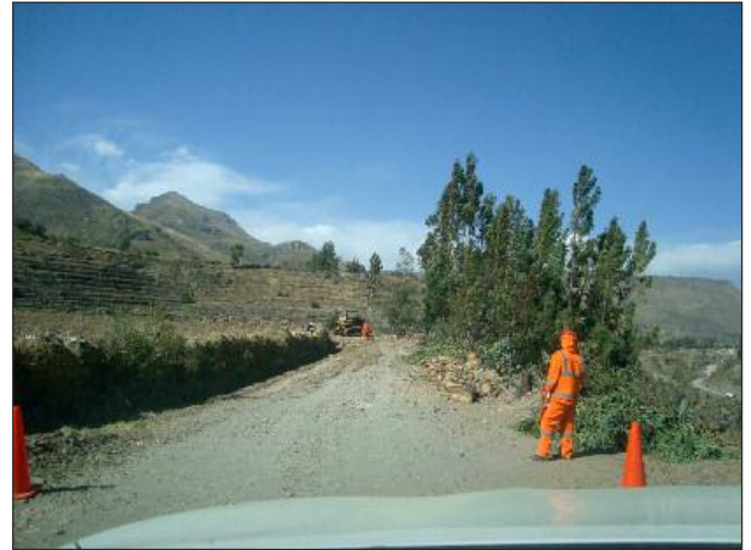
Figure 8. Workmen clearing the road for us to pass.
