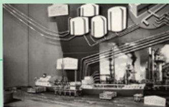
1962 - Egypt - Suez Refinery Terminal
