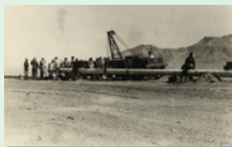
1954 - Egypt - Cairo-Suez Pipeline
