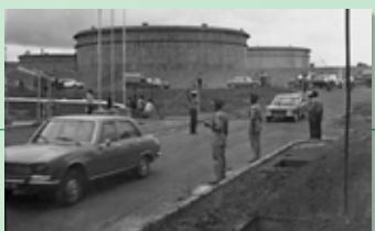
1979 - Nigeria - NNPC Jos Pump Station
