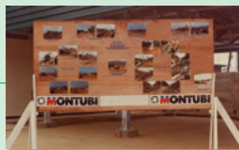
1979 - Nigeria - NNPC Jos Pump Station
