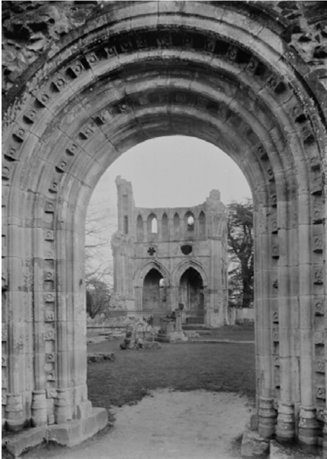
Figure 1: View of the north transept of Dryburgh Abbey illustrating deterioration of carved stone. Crown Copyright: Historic Environment Scotland
