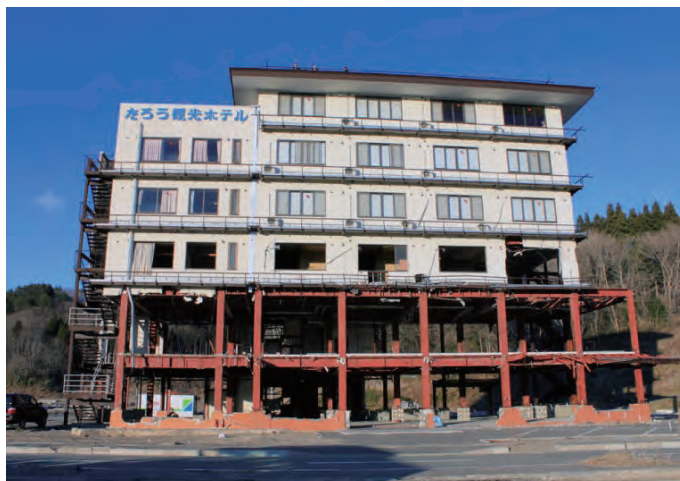
Fig. 9. Taro Kanko (sightseeing) Hotel destroyed by Tsunami preserved as one of the geosites for disaster prevention education in the Sanriku Geopark .
