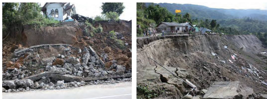
Fig. 4. Landslides triggered by earthquake in Aceh Province on 2 July 2013.
