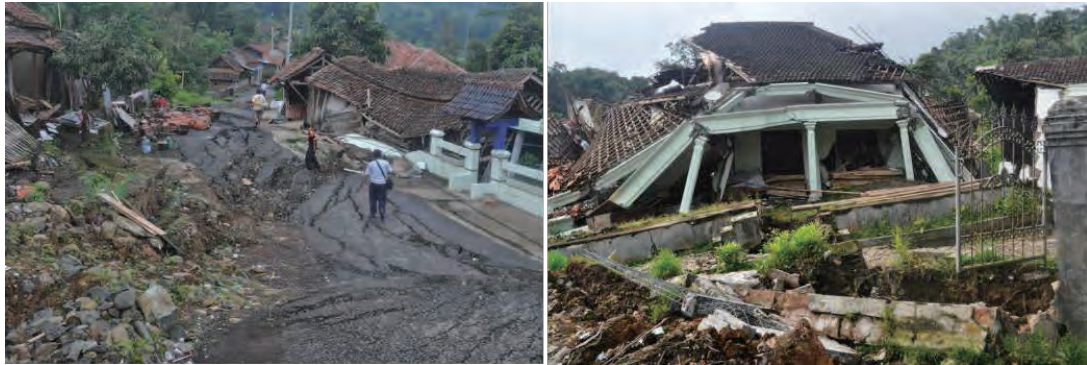
Fig. 5. Houses and road damaged.
