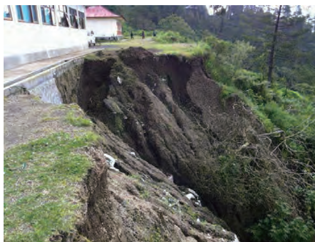
Fig. 2. Condition of school building in Pura Dalem which is still threatened by landslide.
