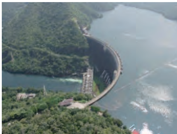
Fig. 10. Water level in upper stream is higher than water level in downstream.
