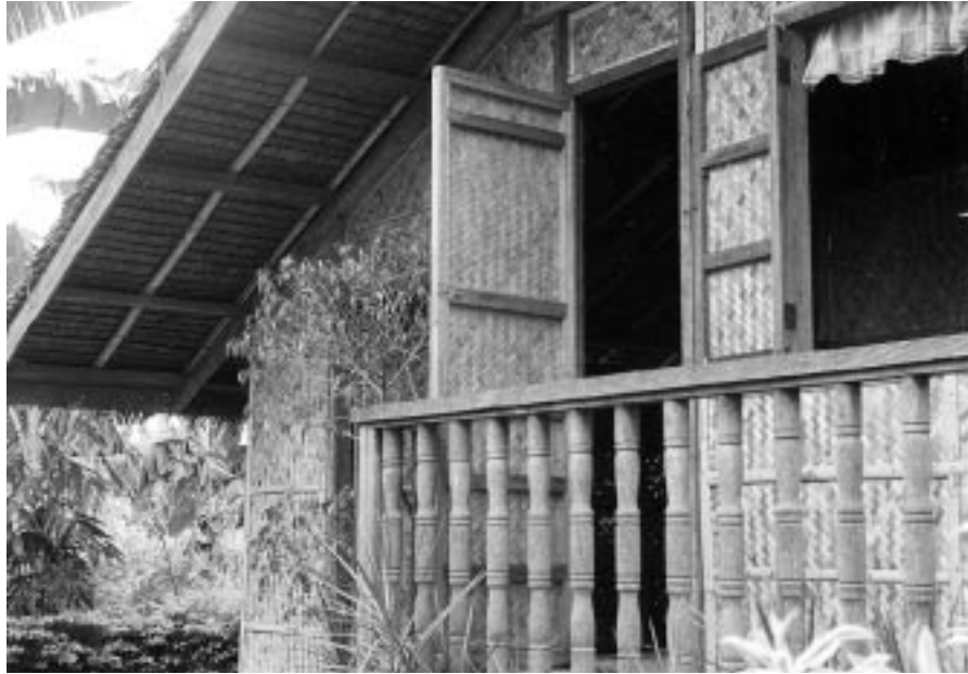
Fig. 1.18. House constructed of coconut palm 'wood' with roof thatch of fronds of Nypa fruticans . Courtesy of Philippine Coconut Authority.
