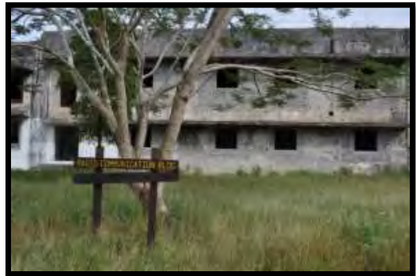
Photo 3.8-7. Japanese Radio Communications Building along Broadway Avenue
