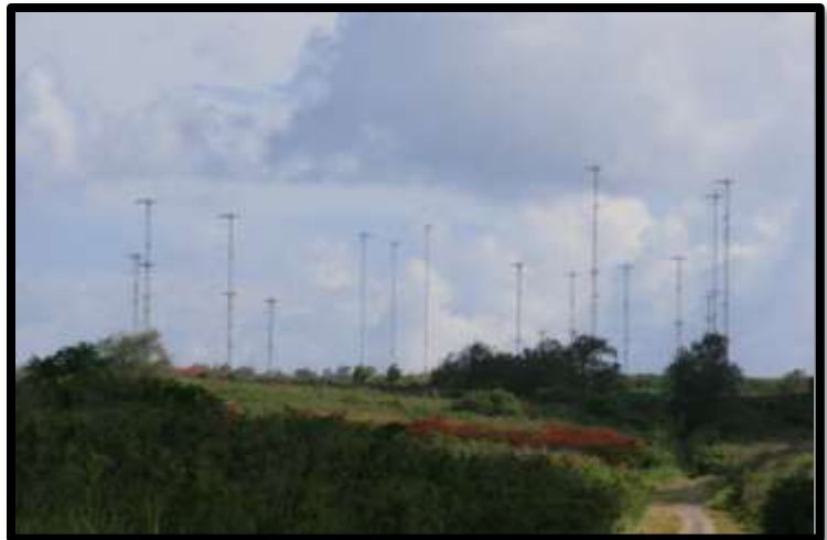
Photo 3.6-1. International Broadcasting Bureau Antenna Array
