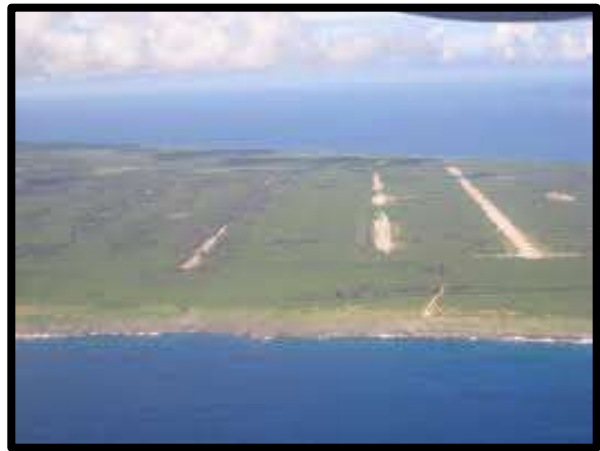
Photo 3.5-1. Aerial View of North Field
