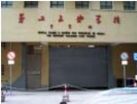
The Workers' Children High School, Macau
