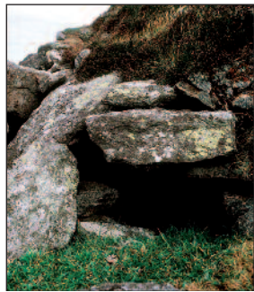
Collapsed broch entrance
