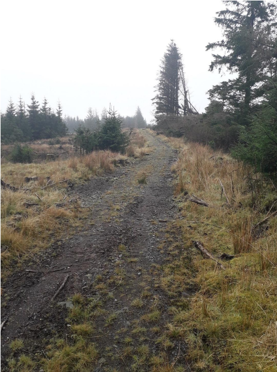
Figure 4 – existing access track east of the proposed borrow pit area
