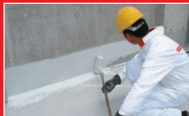
2. 1st Coat of Formak 629
