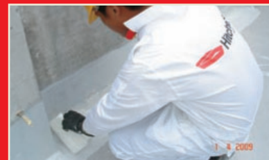
3. Unroll 100mm width fibreglass mat
