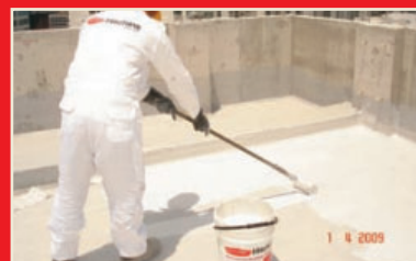
6. Apply 2nd Coat Formak 629 Topcoat
