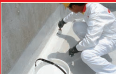
4. Coat Formak 629 over fibreglass
