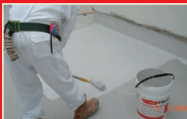
5. Application of 1st Formak Topcoat
