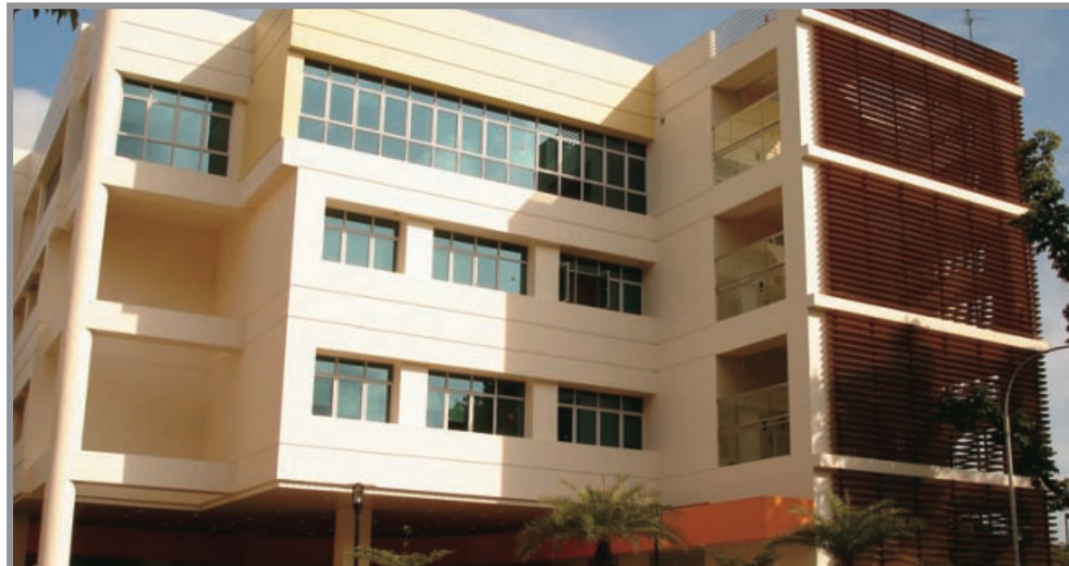
◀ QUEENSTOWN POLYCLINIC - SINGAPORE
