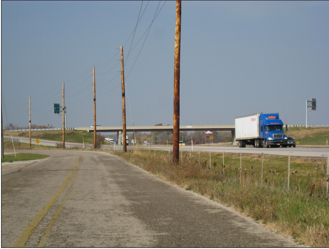
The Fairland Exit Overpass as seen from the Frontage Road looking northwest.
