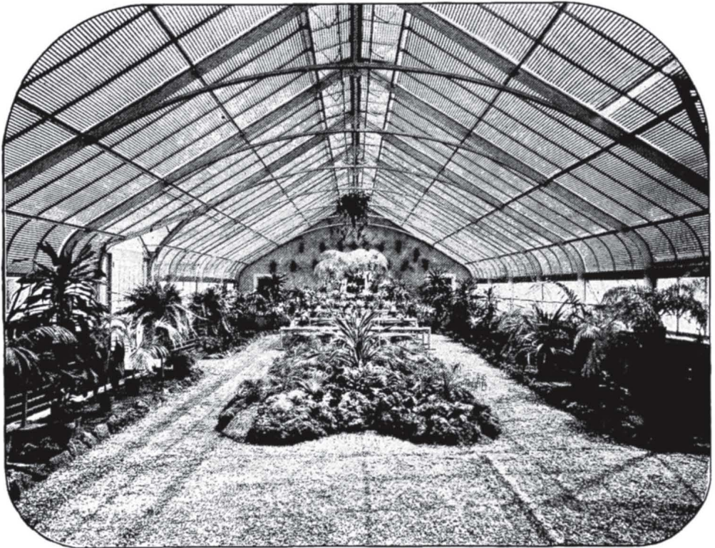
Orchid display house built for Mr. Walter H. Jewell at New Rochelle, New York
