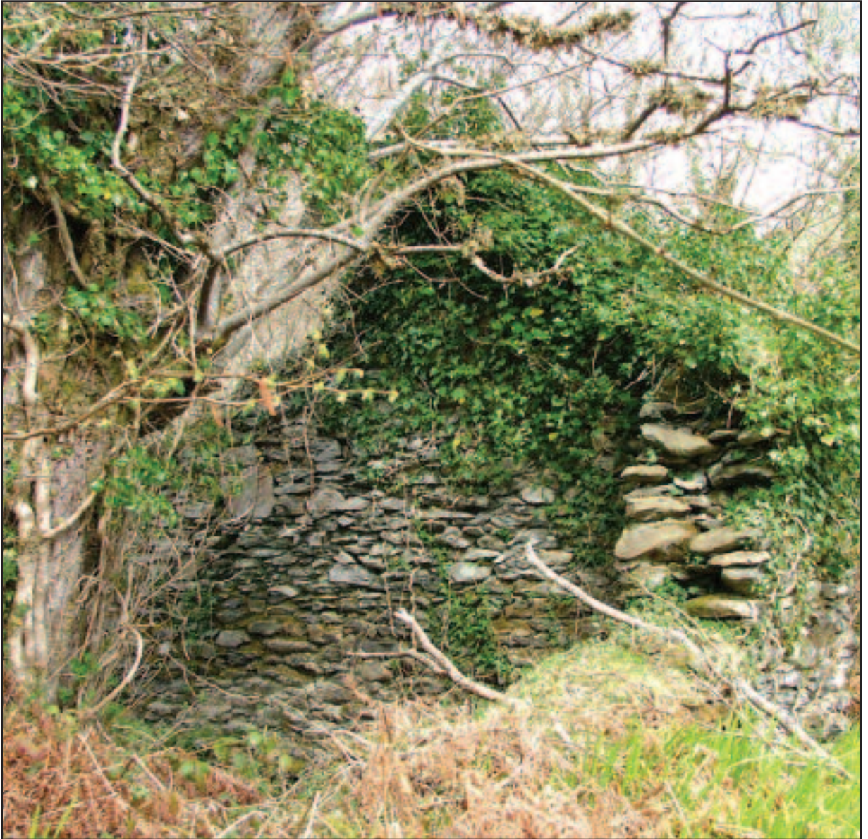
Ruins of wood ranger's cottage.
