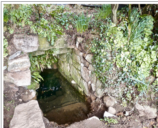
Dipping-well under a hedge at Sancreed. Steps under the water to climb down when the water level falls in summer.
