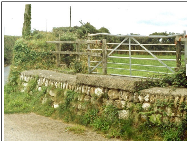
Churn stand built on adapted section of Cornish hedge, which could also be used to off-load fertiliser etc into the field.
