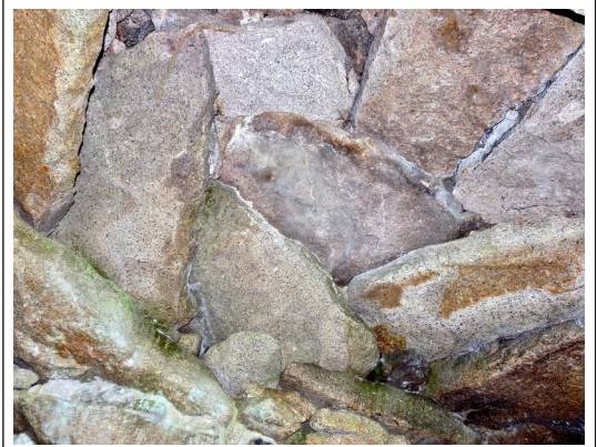
A view looking up inside the crow showing how cleverly the roof was constructed by overlapping flat slabs of granite moor-stone.
