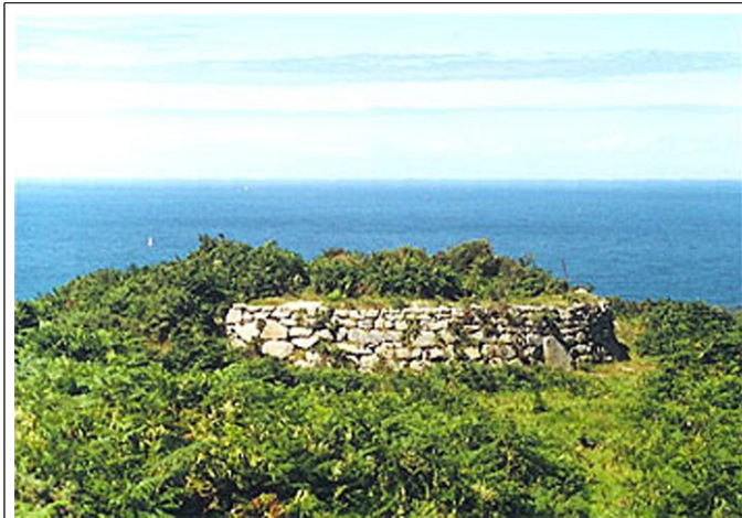
Cornish hedge around mine-shaft.
