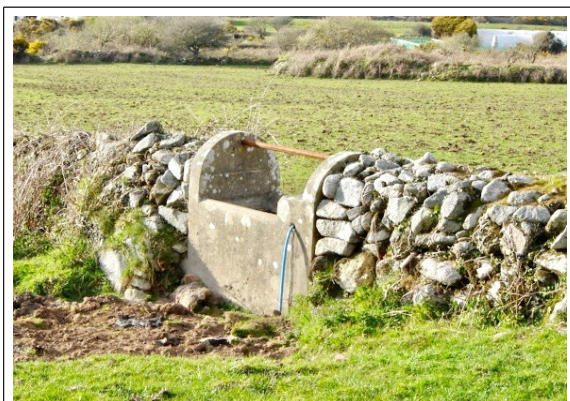
A neat little concrete drinking trough built into a stone hedge to serve both fields.
