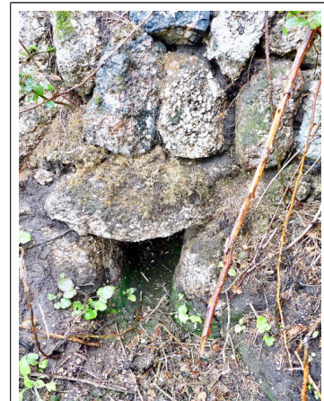
A modest bolt takes a drainage ditch through an old field hedge near St Just in Penwith.
