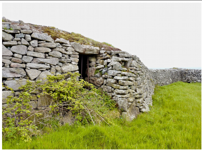
Pig's crow built into a massive stone clearance hedge in West Penwith.
