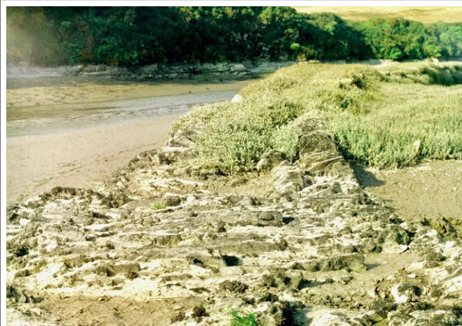
Slate-built Cornish hedge enclosing pool for tide-mill on the river Camel, now disused. Foreground section breached by the sea since maintenance discontinued shows remains of basic construction.
