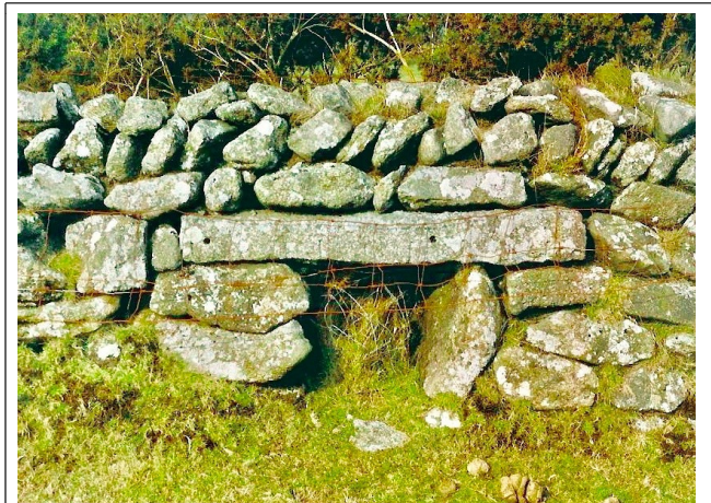
Sheep-creep on Bodmin Moor. The lintel is typical of stone that had been destined or used for some other purpose before being built into the hedge - in this case a redundant gatepost, showing the two holes drilled to take hinge crooks.
