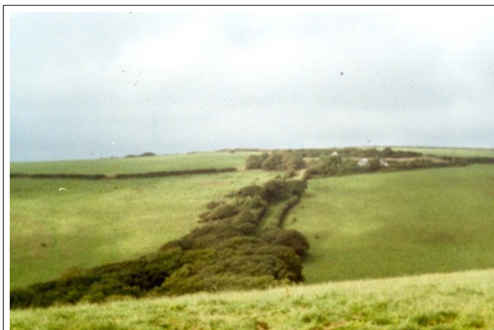
Bude canal incline at Hobbacott Down, with the position of the pumping-house at the top clearly identifiable. Its parallel bounding hedges are visible though partly overgrown by scrub.
