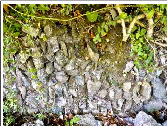
Typically poor and neglected smallholding hedge built of broken mine spoil, dividing fields to a miner's cottage of 1820, near Hayle.
