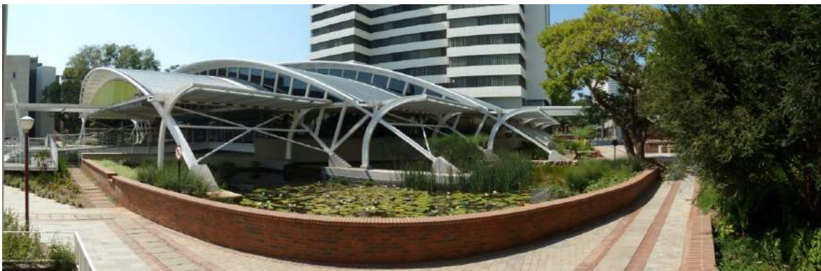
Fig 10, the South-western shallow pond of the rainwater harvesting pond as seen from the entrance to the Engineering 2 labs. Photo: Neal Dunstan.
