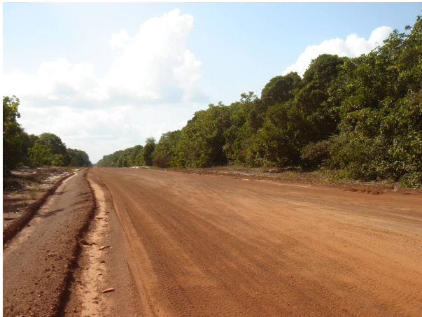
(c) Dakama forest (right of road) may develop as a on white sand. This may resist further degradation, but comprises only small trees. The soil is white sand, with the laterite on the road bed being artificially laid.
