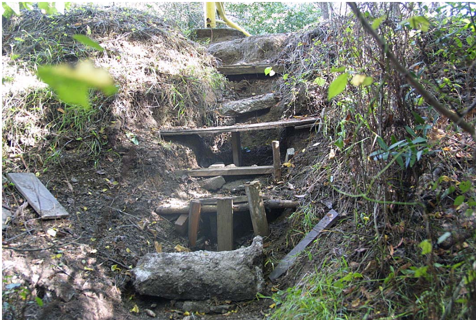
Figure 7 Hiker-built steps across an eroding gully lead to a social trail under the redwoods
