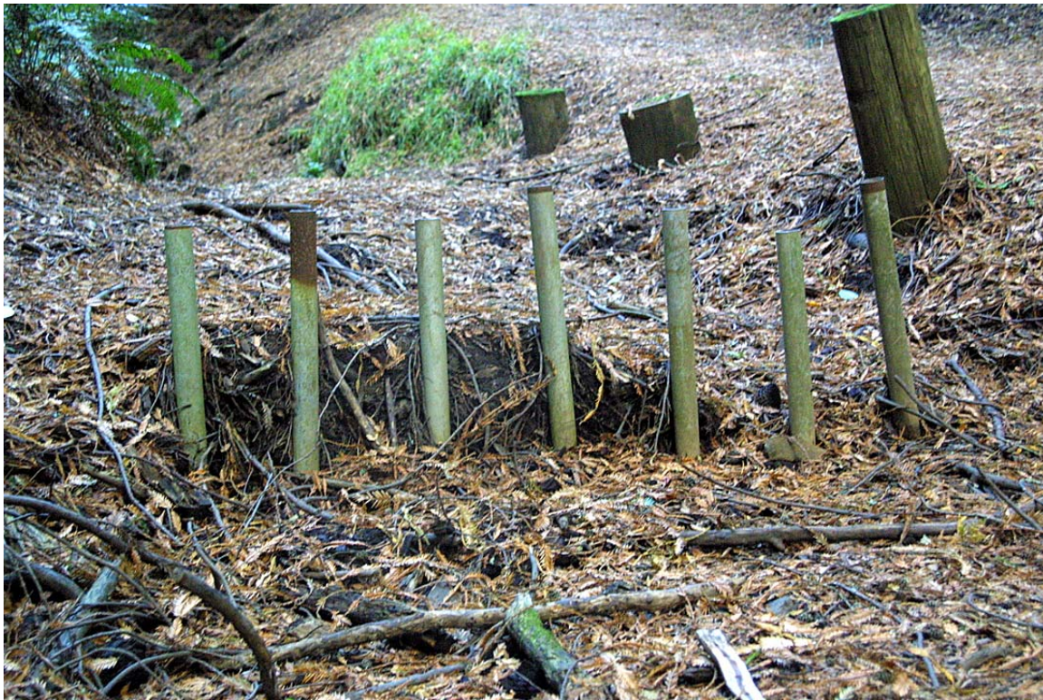
Figure 13 Weir traps sediment at hump upstream, diverts flow to the right
