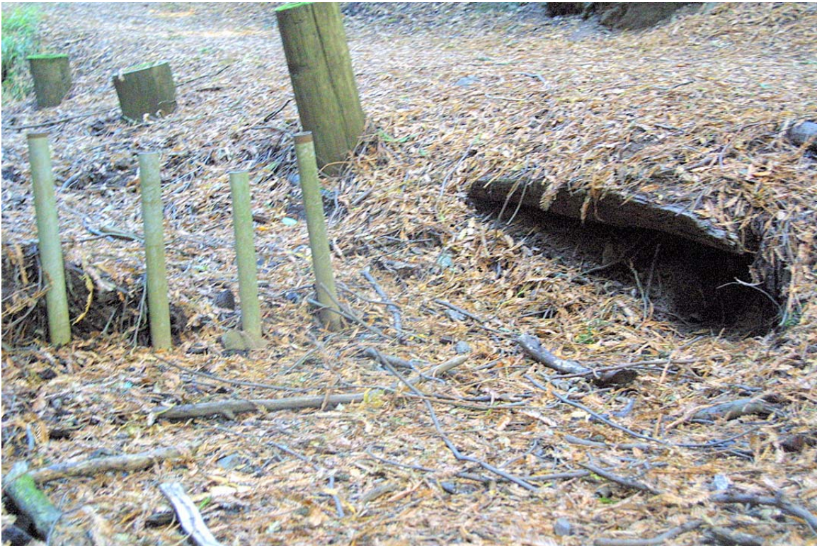
Figure 14 Diverted flow from weir undercuts trail
