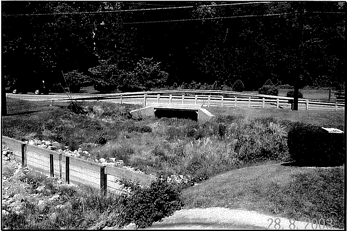
Photo 7. Area 4 with Data Point #3 located near the center of the photo. The adjacent drainage swale is visible coming in from the right. Notice the detention weirs.
