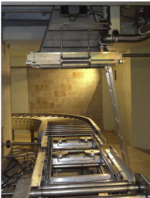
Figure 1.13 Scan horn and conveyor system of an Iotron IMPELA® 10/50 Linear Electron Accelerator Installed at Iotron Industries USA Inc., Columbia City, Indiana (photo courtesy of Iotron Industries Canada/USA Inc.). For color version of this figure, the reader is referred to the online version of this book.
