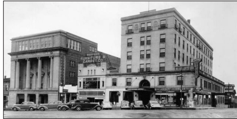
The Greystone Hotel is shown here anchoring the corner of the north side of the Bedford square. The grand hotel was a southern Indiana landmark from 1923 until it fell to the wrecking ball in 1994.
