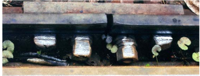
Check-Rail on worn inner Curve Rail with Check-Rail Block and Pandrol-Fast-Clip on Trough Steel-Sleeper. Wheels riding on the Check-Rail Blocks and Wheels cutting into the Fishplate Bolts.; Hatton Section, Rozella
