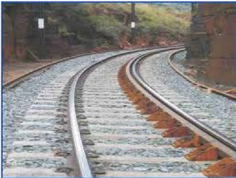
Curve Check-Rail with Pandrol Bracket-Fastening and e-Clip Rail-Fastening in South-Africa
