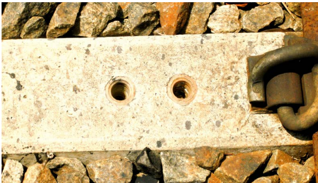
Dowels in Concrete-Sleepers for Indian Check-Rail Bracket-Fastening
