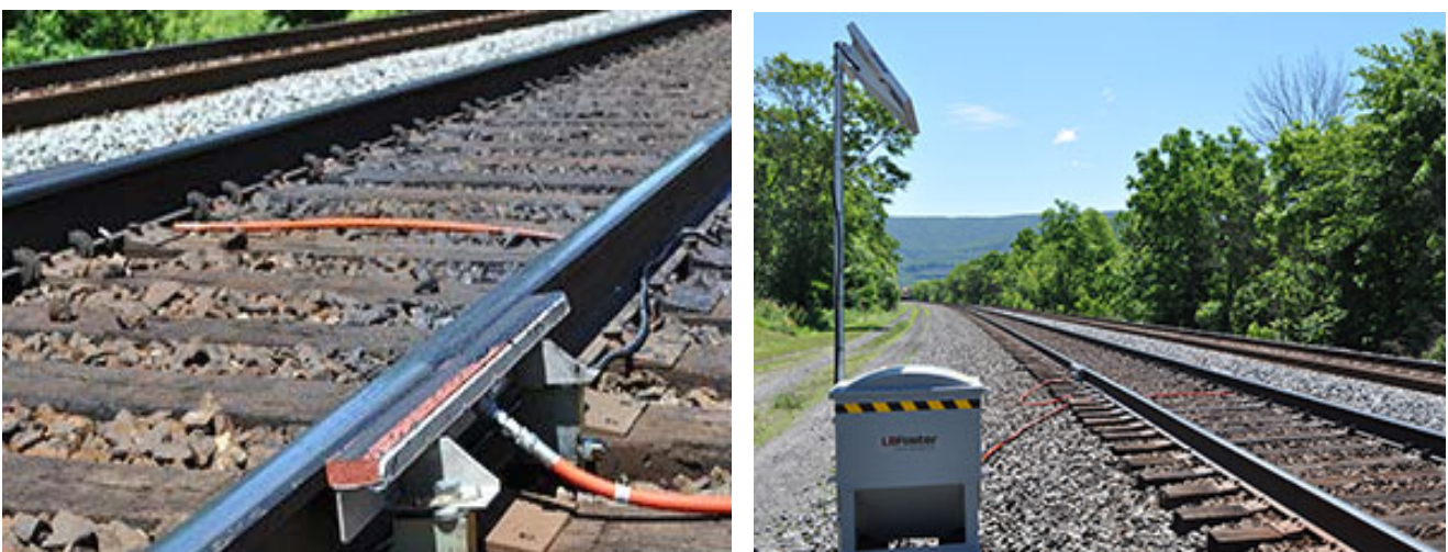
Automatic Wayside Top-of-Rail Lubrication with a Friction Modifier, LB Foster
