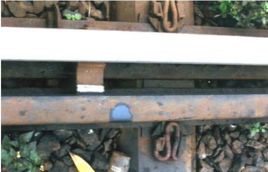
Check-Rail on worn inner Curve Rail with Check-Rail Block and Pandrol-Fast-Clip on Trough Steel-Sleeper. Wheels riding on the Check-Rail Blocks and Wheels cutting into the Fishplate Bolts.; Hatton Section, Rozella
