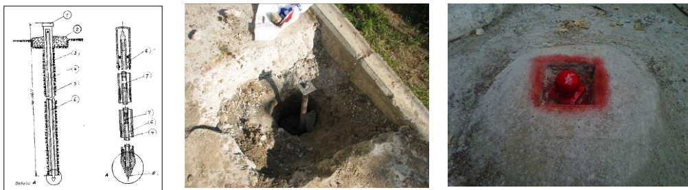
Fig. 4 The mounting of the reference depth benchmarks
