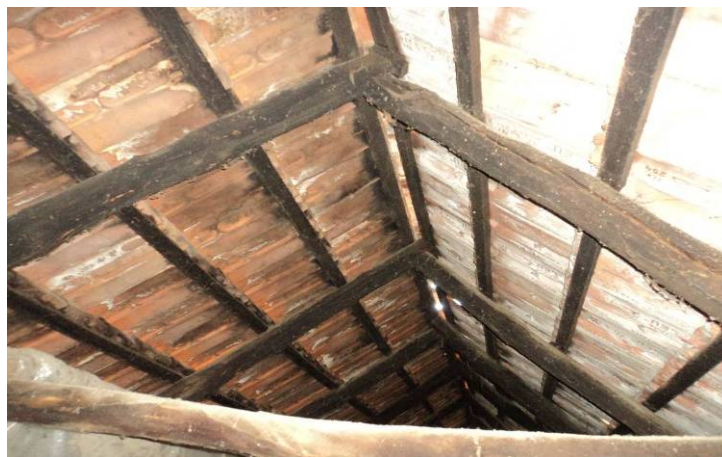
Fig. 4. The framing of the roof
