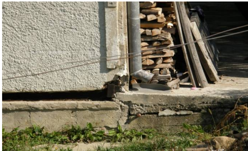
Fig. 3. Sidewalks Distancing from House Walls (Fulău Dumitru).
