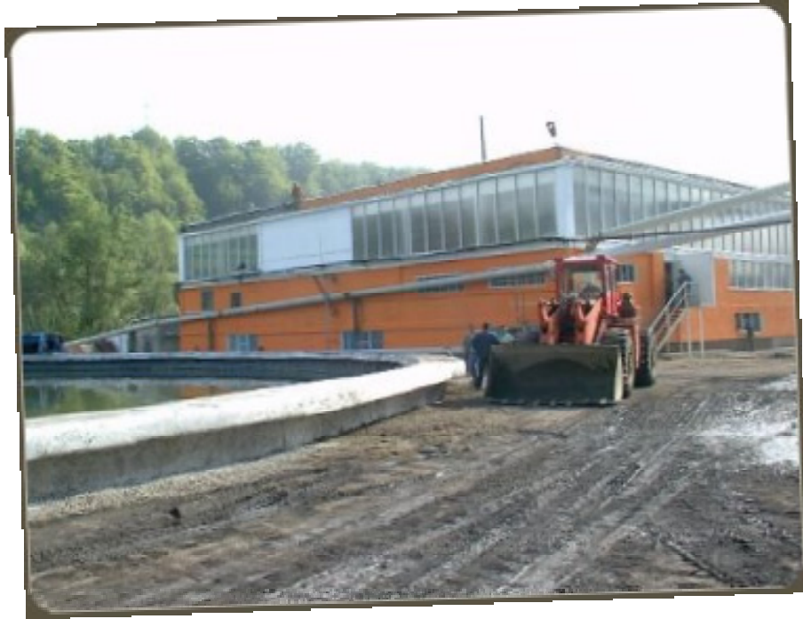
Fig. 1 Settling pond at Coroiesti treatment plant [1]
