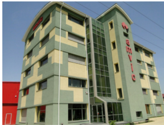
Fig. 8 Passive office building AMVIC – Bragadiru
