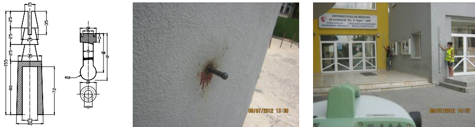
Fig. 5 The observation marks, on the inside and on the outside of the buildings
