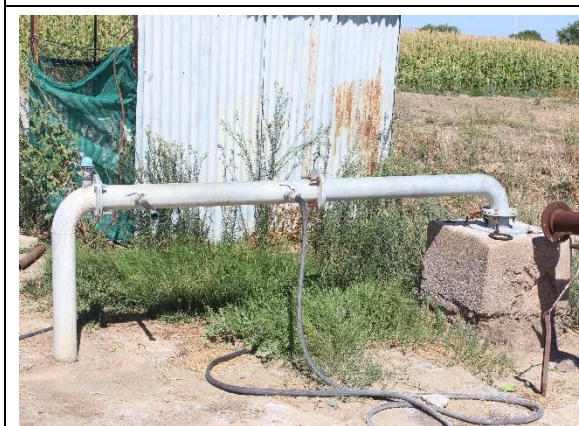
Photo 4-11 Borehole with installed pump
