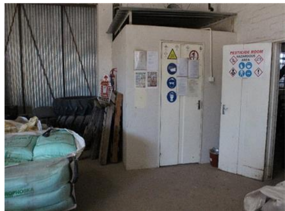
Photo 4-16 Chemical storage area
