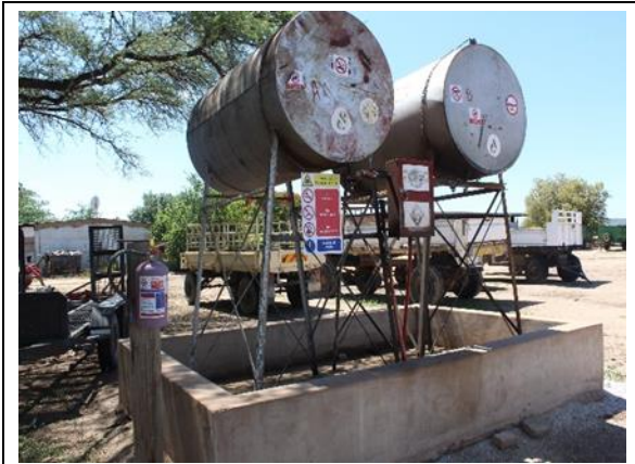
Photo 4-13 Consumer fuel installation
