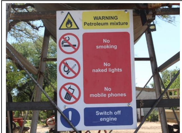
Photo 4-14 Warning signs at fuel storage
