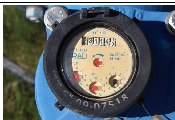
Photo 4-10 Flow meter at irrigation boreholes
