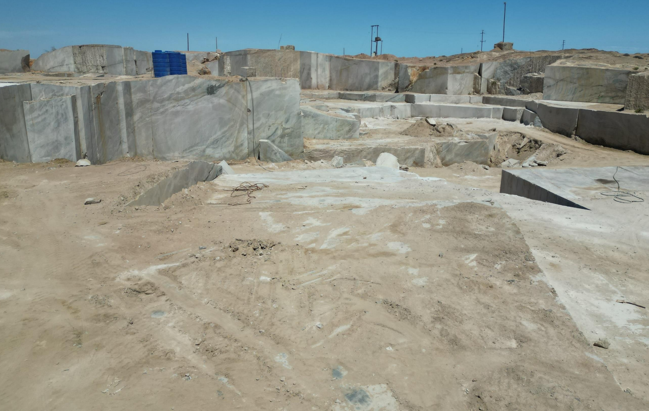
Plate 2.4: Drone image showing the southwestern view of a working / extraction face at a granite quarry in the ML No. 123.
