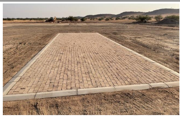
Photo 3-12 Interlocked slab
