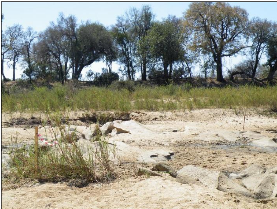
Figure 2-4 : KCP View from left bank end of rock sill to right bank.
