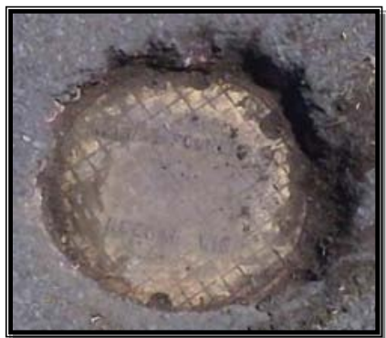
Figure 5.3 Two Typical Borehole Plate Covers commonly found in the middle of Municipal Streets and State Highways throughout the Coal Fields (Photos taken by Robert E. Hughes, EPCAMR, 2011)
