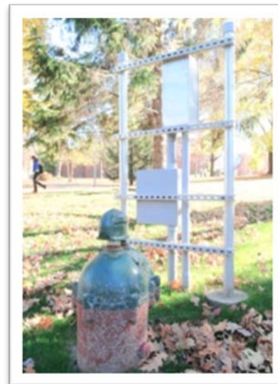
Figure 2. Explaining Marywood's Geothermal Energy Usage by Kevin O'Neill-Staff Artist for The Scranton Times Tribune and Photo by Linda Morgan / Staff Photographer-The Scranton Times Tribune A wellhead outside Marywood University's School of Architecture is about all that's visible of the geothermal system (Tribune, 2010)
