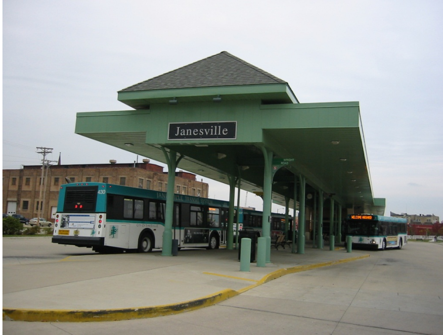
Figure 3: An Example of Sawtooth Berthing at a Transit Center
