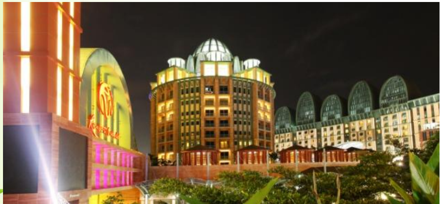
Project Name: Resorts World Sentosa Landscape Drainage Specialist: Fast Flow Singapore Pte Ltd
