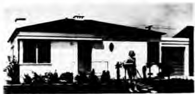
California has proved a fertile field for Title I, Class 3 (new-home) loans, since the climate facilitates building of homes within the $2,500 loan maximum
