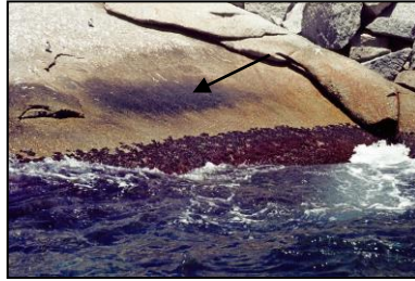
Fig. 1: slippery, dark-stained granite rock (arrowed) in a zone that is wet from wave surges, at Victor Harbor, SA
