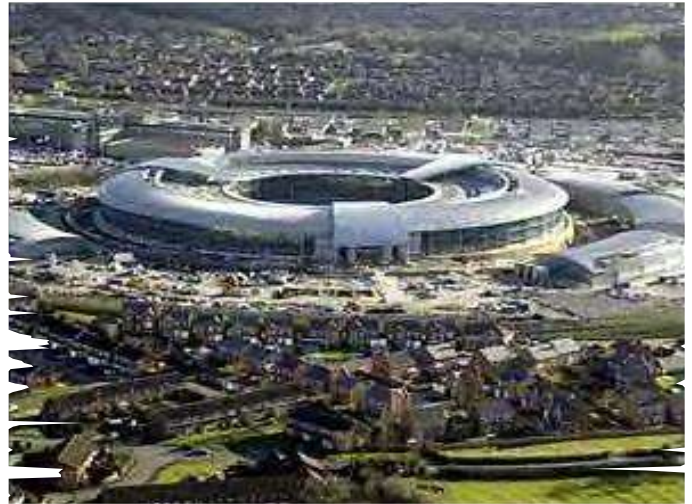
HEADQUARTERS AT BENHALL, CHELTENHAM
